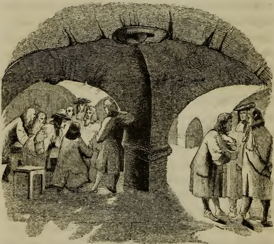
VAULT UNDER HURLEY-HOUSE.
